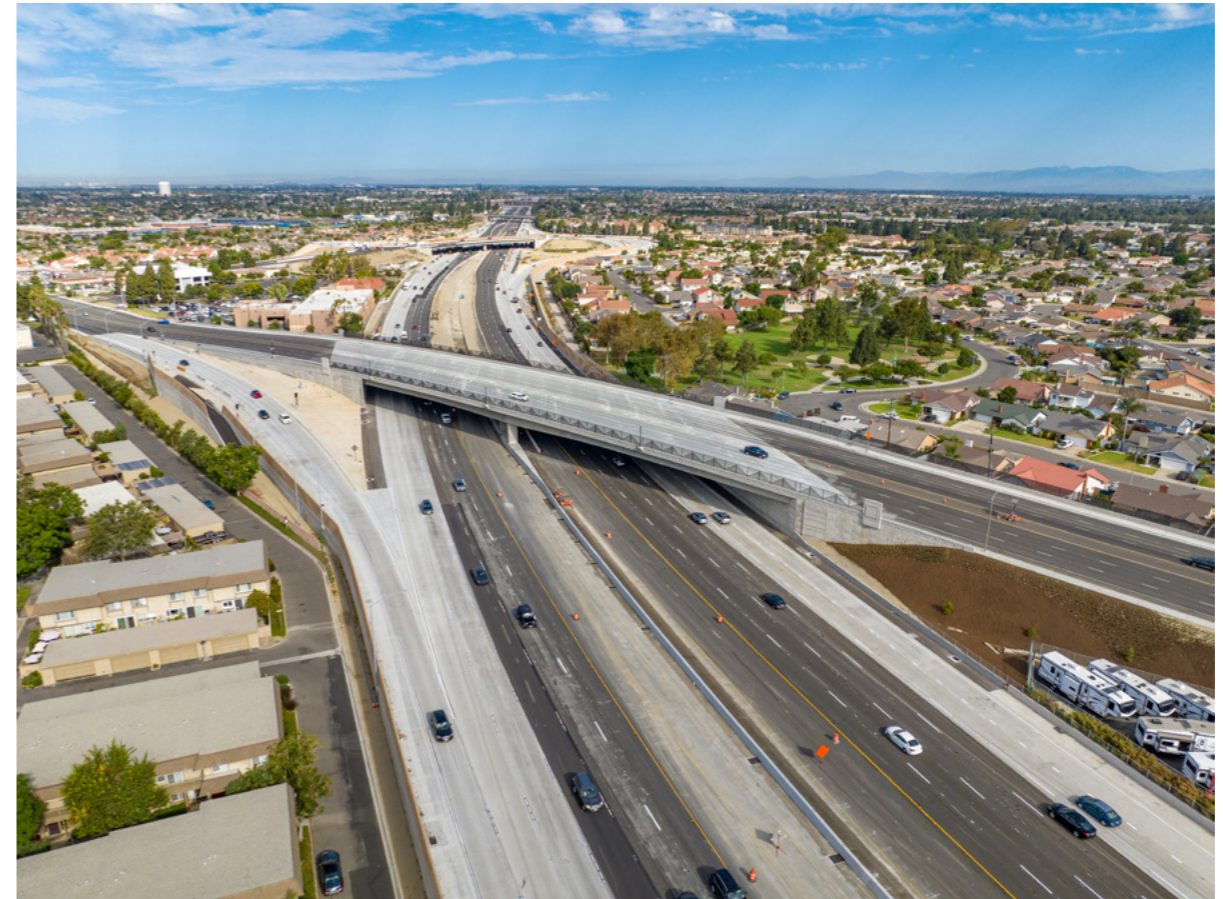
I-405 improvement project. California, USA.
