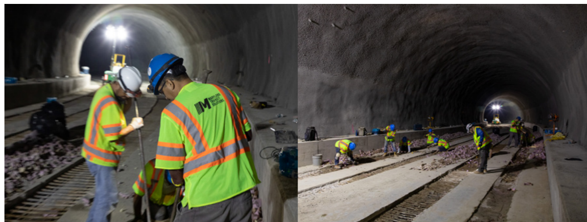
Purple Line. Maryland, USA.
