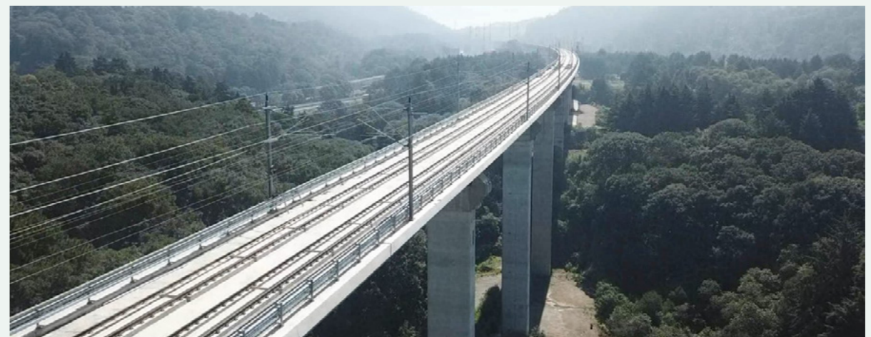
Viaduct 2, Mexico City-Toluca commuter rail. Mexico.
