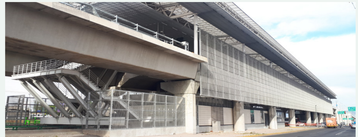
Zinacantepec station, Mexico City-Toluca commuter rail. Mexico.
