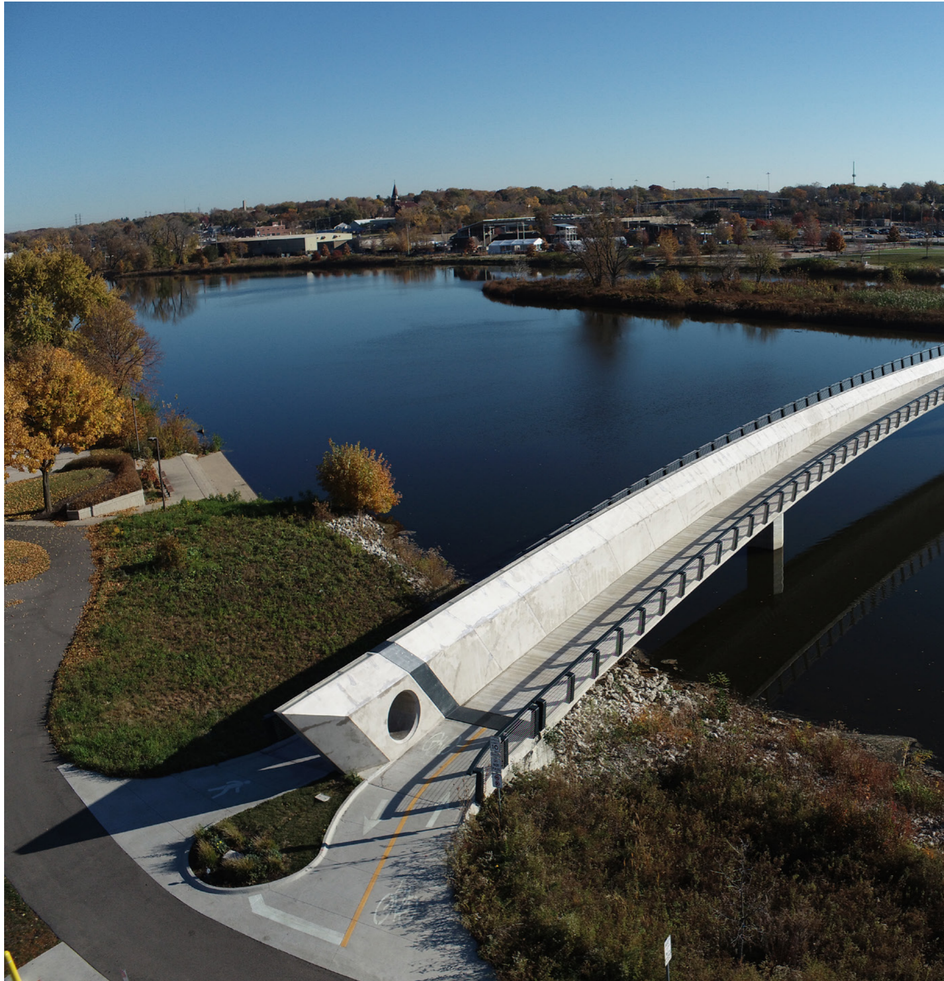
Puente peatonal Aurora Transportation center. EEUU.
