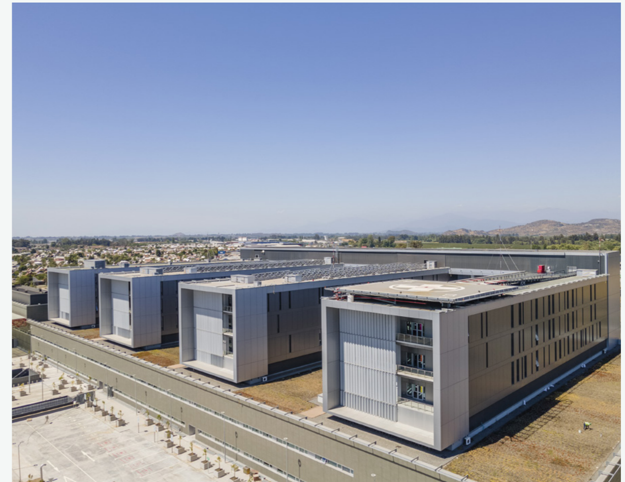
Hospital de Curicó, Chile. CES 2022 award – Sustainable Building.
