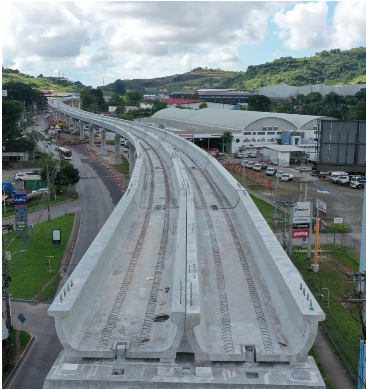
Rail viaduct. Metro Line 1 extension project, Panama.
