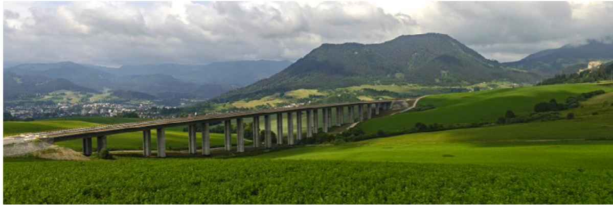
Hubová-Ivachnová section of the D1 motorway. Slovakia.
