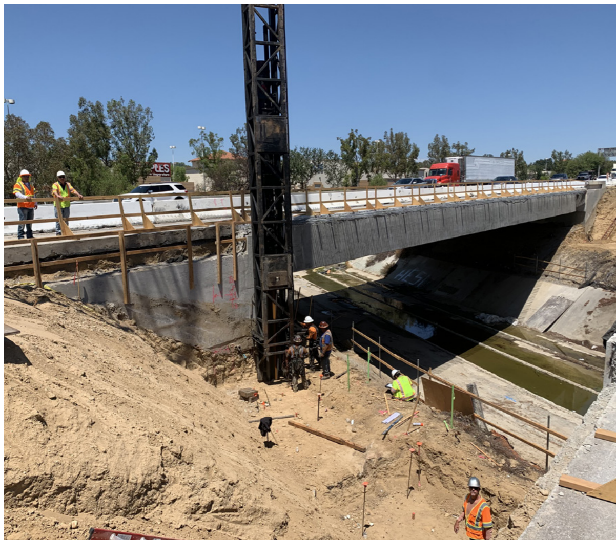
I-5 capacity improvement project. Los Angeles, USA.
