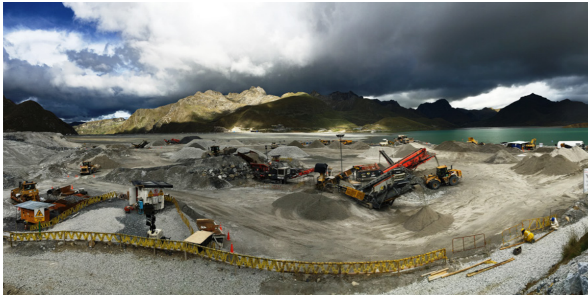
Tailings dam. Antamina mine. Ancash, Peru.
