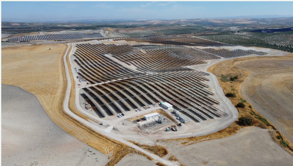
50 MW photovoltaic plant, Olivares, Jaén, Spain.
