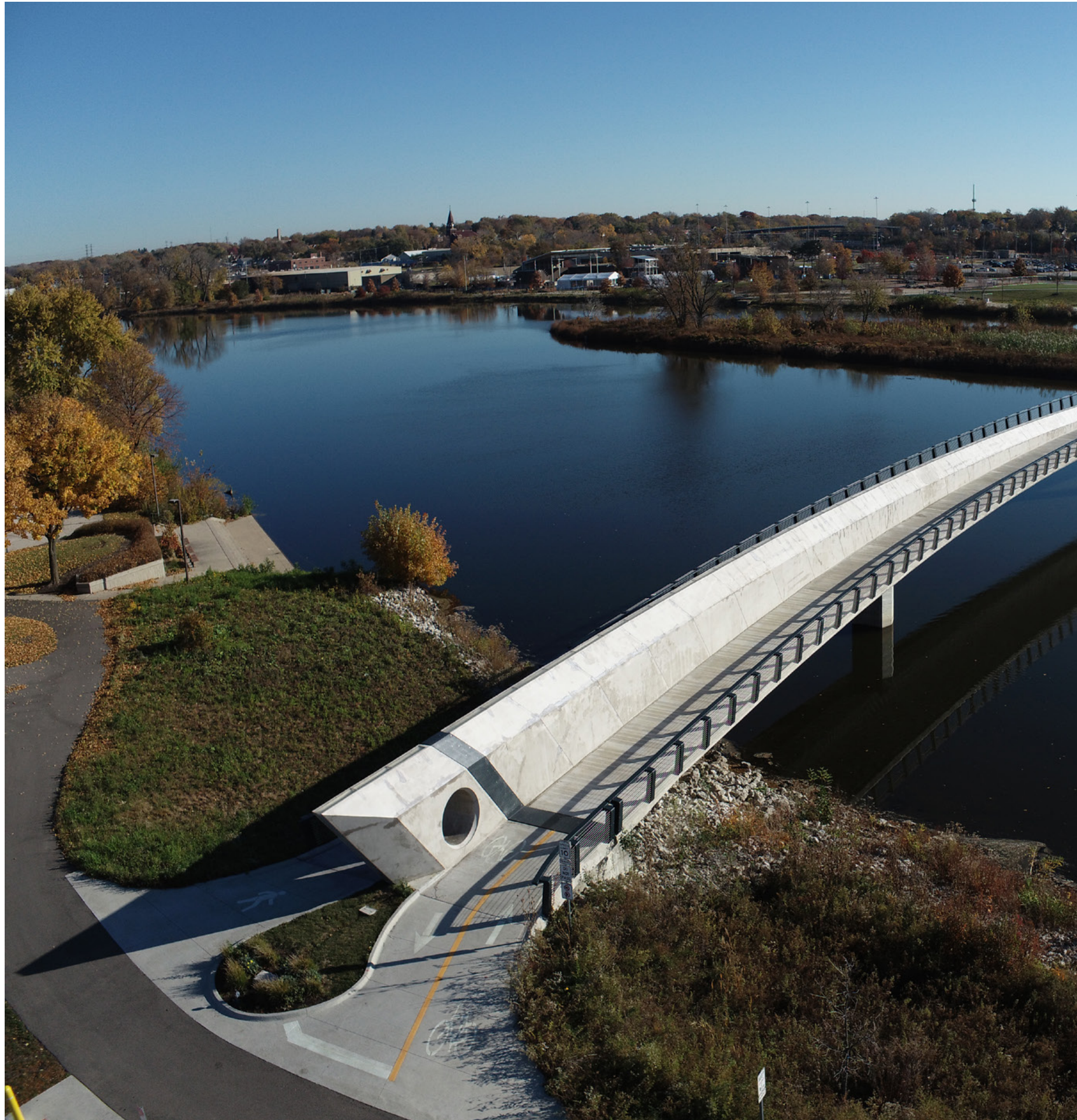
Puente peatonal Aurora Transportation center. EEUU.
