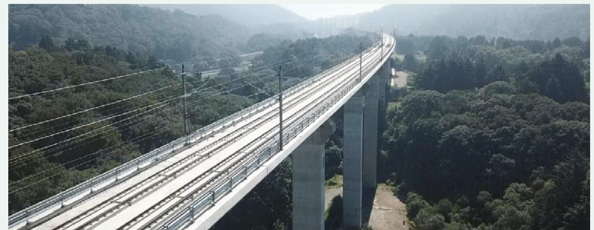
Viaduct 2, Mexico City-Toluca commuter rail. Mexico.
