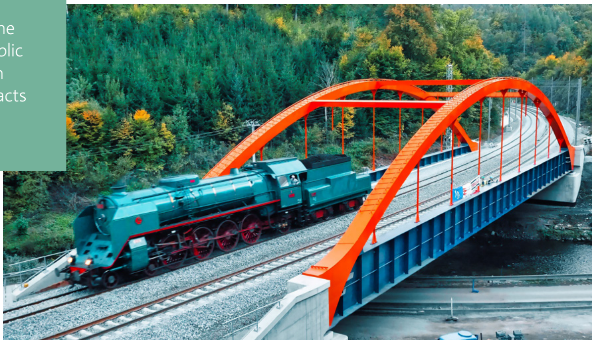
Reconstruction of the railway bridge over the Svitava River. Czech Republic.
