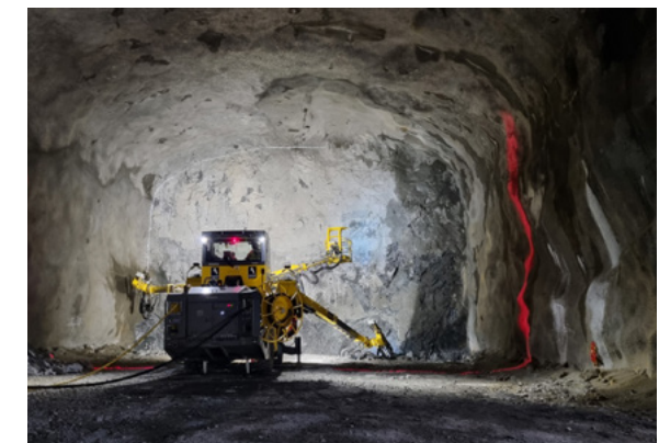
Extension work on the Stockholm Metro Blue Line from Gullmarsplan station. Sweden.
