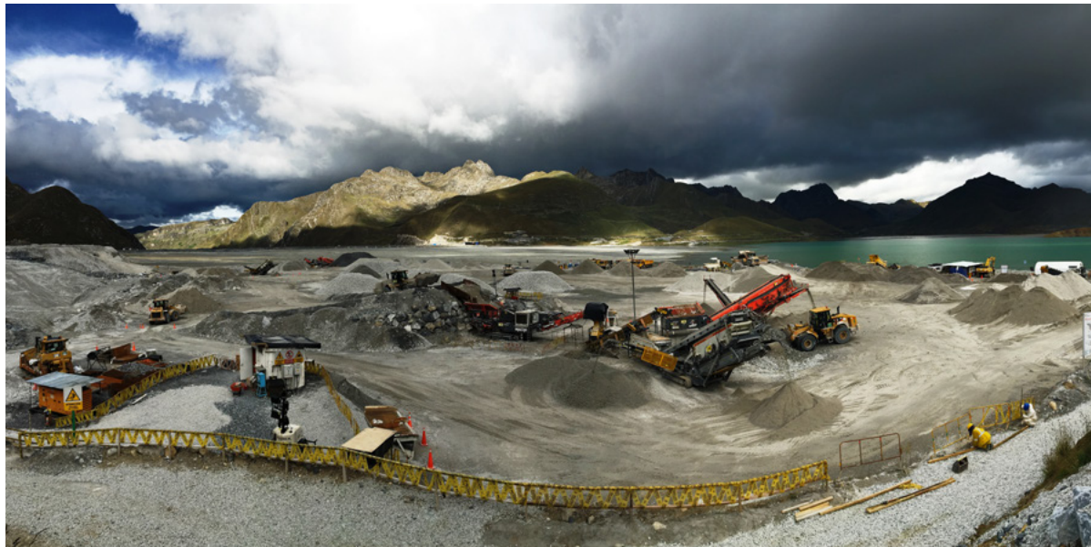
Tailings dam. Antamina mine. Ancash, Peru.
