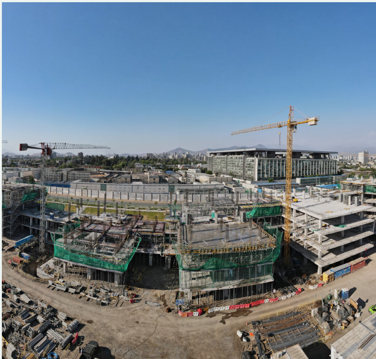
Construction of Forensic Medical Department. Santiago de Chile, Chile.
