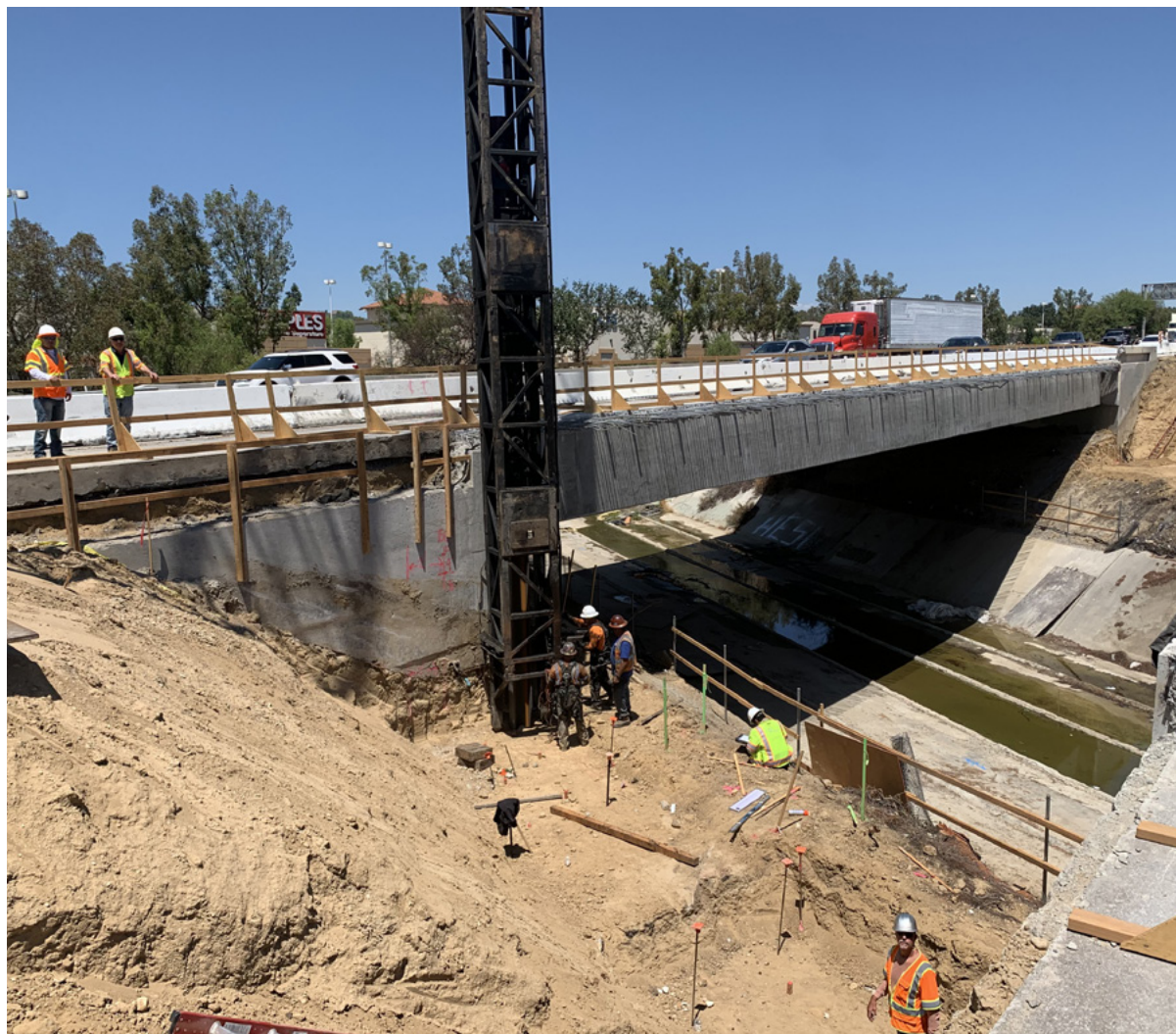
I-5 capacity improvement project. Los Angeles, USA.
