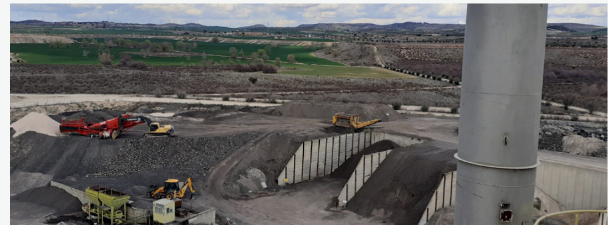
Recycled aggregate plant in Arganda del Rey, Madrid, Spain.
