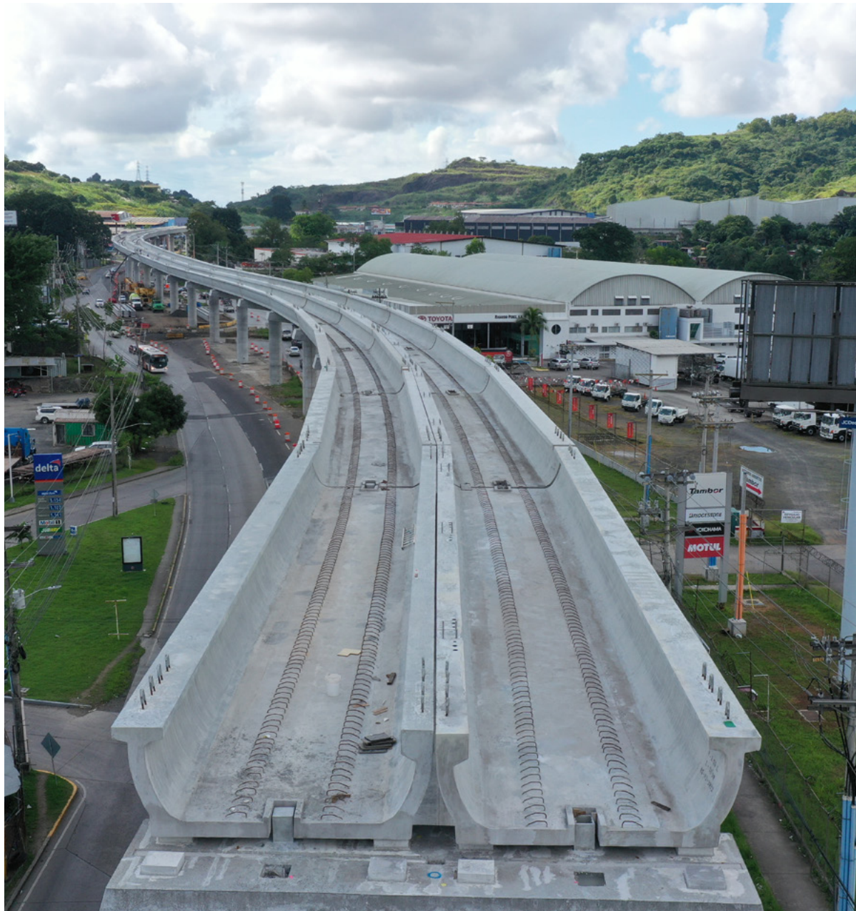
Rail viaduct. Metro Line 1 extension project, Panama.
