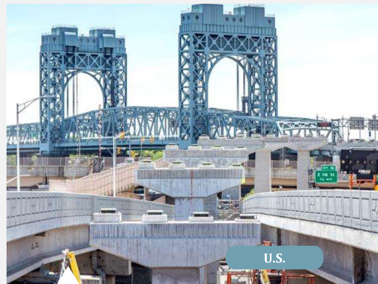
Robert F. Kennedy Bridge Connector Ramp. New York
